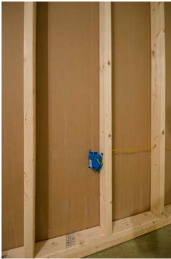
Figure 14: Detail of electrical box on back of wall
