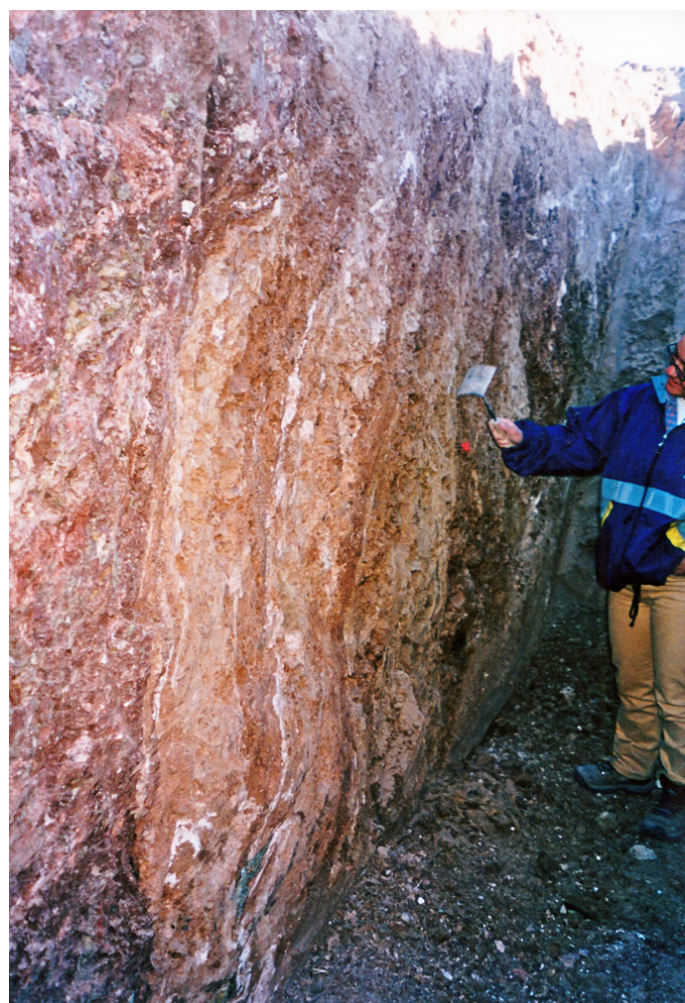
Figure 11. General view of Trench-4. Strongly sheared units and vertical sliding surfaces are seen clearly.
