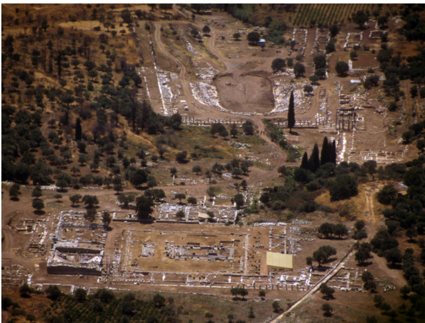
Figure 2. Aerial view of the Asklepion (below) and the Stadium (above) from Acropolis
