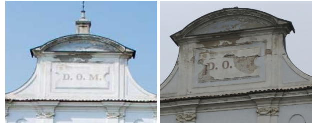
Figure 6. The upper part of the façade before (left) and after (right) the earthquake.
