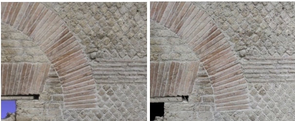
Figure 4. Visual comparison between the Photogrammetric mesh model (left) and the coloured scanner point cloud (right). It is interesting to point out that the density of the point model is so high that the difference between the laser and the photogrammetric model is almost irrelevant, allowing to clearly distinguish every details of the façade on both models
