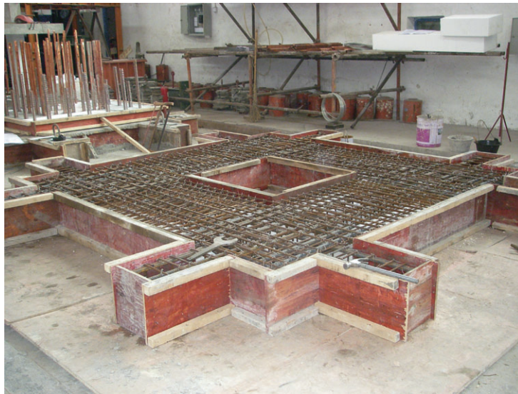
Figure 6. Base beam construction.
