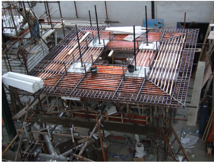
Figure 7. Steel beams and trusses assembling at roof level.
