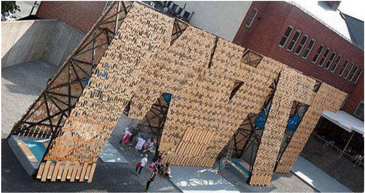
Party Wall , in the courtyard of MoMA PS1 in Long Island City, made from recycled steel and skateboard wood. photo / Zachary Tyler Newton
