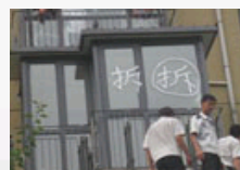
楼下露台搭棚封顶侵权
