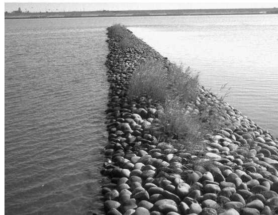
Photo 1 Stable flow around spur dike
