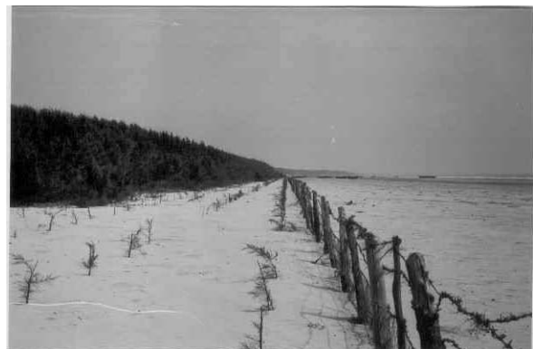
Fig. 3 Bamboo and wire fencing in the neodune area to protect the plantation on bare supratidal beach
