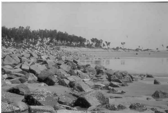
Fig. 2 Revetments boulders used for beach protection thrown away from their original positions and strewn haphazardly on the beach. Many boulders act as hard substratum for the settlement of barnacles and oysters
