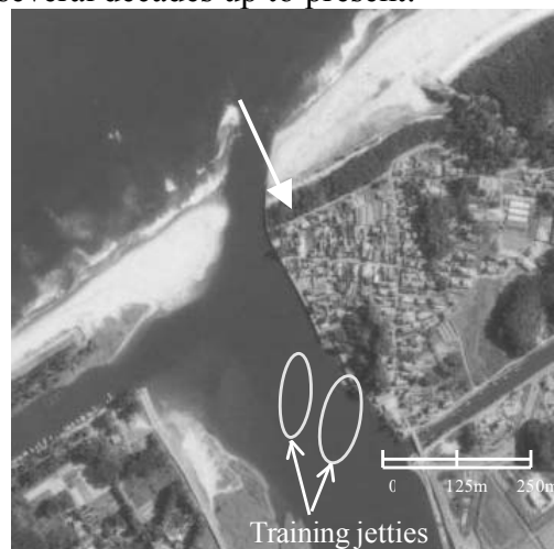
Photo 2 Sediment deposit between jetties(Jun.14, 2002)
