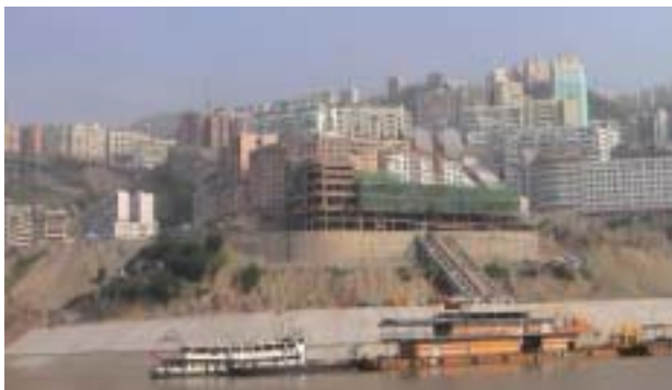
图 1 奉节县新城三马山主城区 Fig.1 Sanmashan urban area of New Fengjie County
