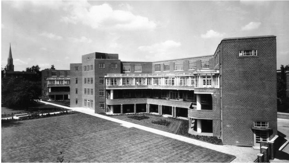
Figure 3: The private patients' block at the Maudsley photographed in July 1939. It was designed by the LCC architects E P Wheeler and G Weald. It had an enclosed roof garden for patients who were thought likely to harm themselves (London Metropolitan Archives).
