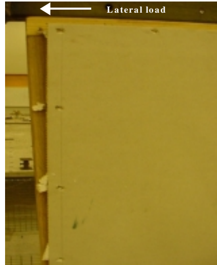
Fig. 4 A photo of a top corner of Wall 1 at displacement of about 35mm showing deflected shape of the end stud and failed plasterboard nail connections.
