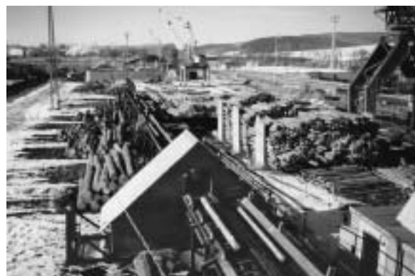
Figure 1 The entry of a cross-cut and sorting line in the Bylnice sawmill in the period of measurements (the scanning device is placed in a wooden shelter)
