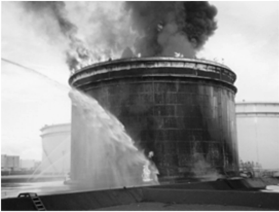
Fig. 4 Tank fire just after the earthquake (photo by Tomakomai Fire Service).
