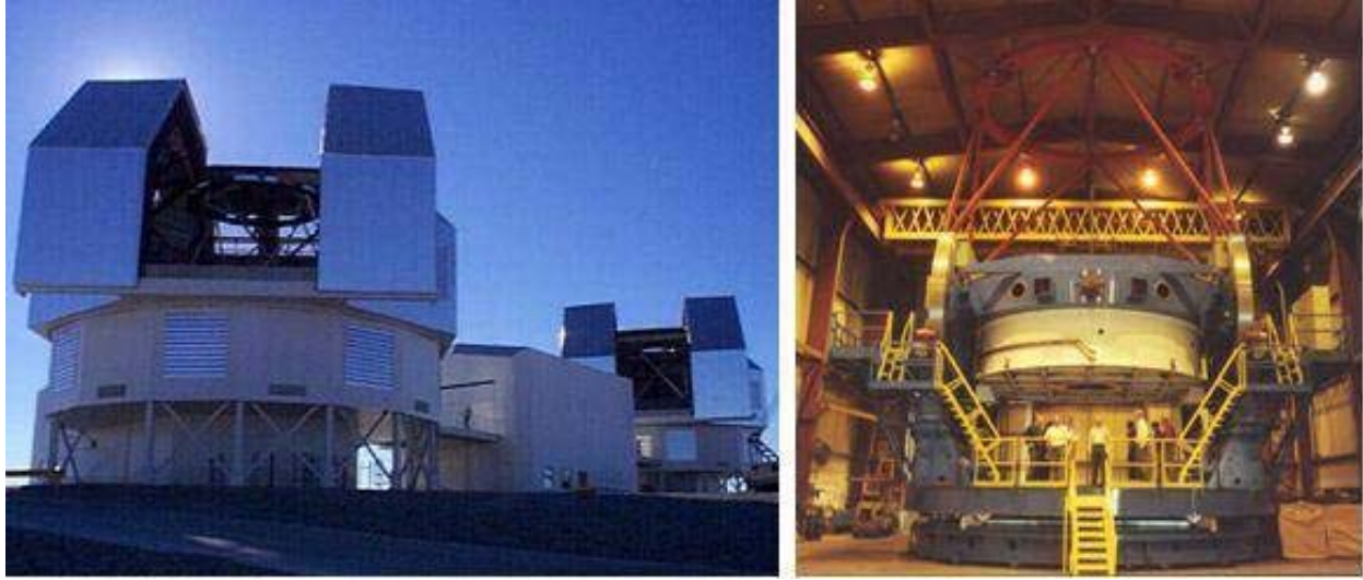
Fig. 5. The Magellan telescopes in operation at Las Campanas (left panel), showing the housing and common facility buildings. The right panel shows the telescope structure at the L&F factory.
