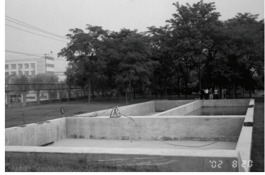
FIGURE 6: Photo of the recharge pool.
