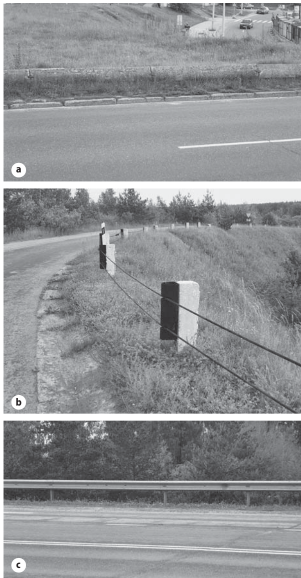
Fig. 4. Guardrails installed on highways: a – reinforced concrete guardrail; b – cable guardrail; c – metal guardrail
