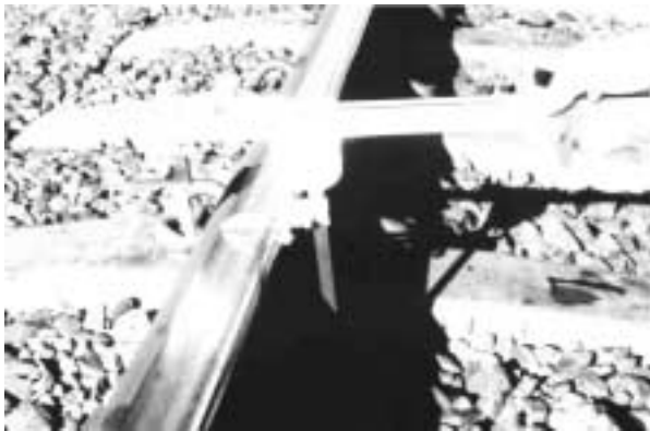
Fig 1. Side wearing measurement on the curve No 4
