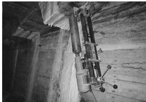
Fig 10. Special coring equipment for inspection of prestressed tendons and their ducts
