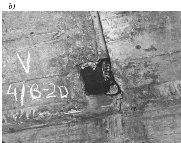
Fig 13. Corrosion of exterior anchors of tendons: a) – at the edge of simple beam; b) – at the joint of segmental post-tensioned bridge beam
