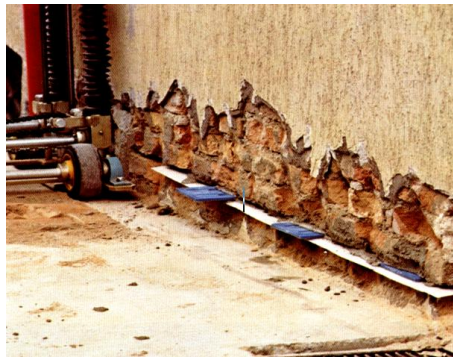
Fig. 3. – Placing wedges into the slot.
