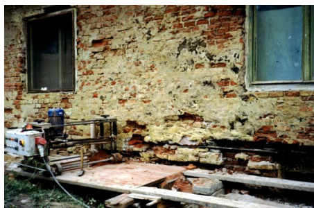
Fig. 4. – Previously described method applied on a brick wall.
