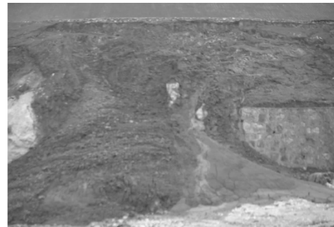
图2 红粘土边坡滑坡 Fig.2 Landside of red clay slope
