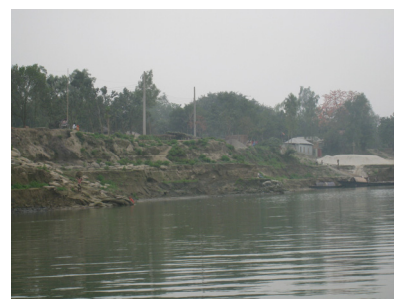
(b) Erosional point at Sirajganj (bank sliding occurred for downcutting of river bed).
