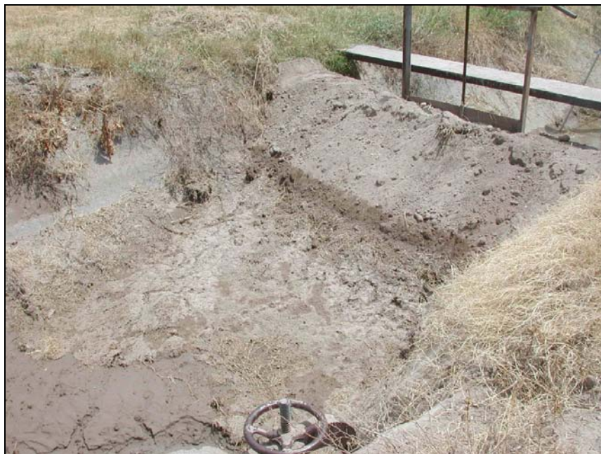
Figure 5. Upstream dam of Test Segment MA4.
