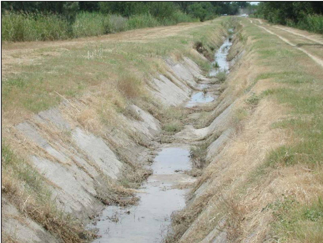
Figure 2. Test MA4, a segment of the lined canal Lat. 2Ac.
