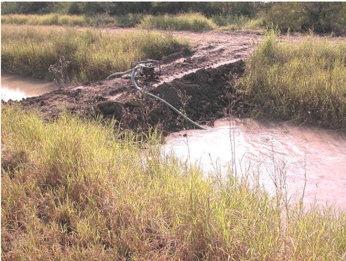
Figure 3. Upstream test dam and the centrifugal pump (a 3-inch "gator-pump") used to fill the test segment to normal operating depth.
