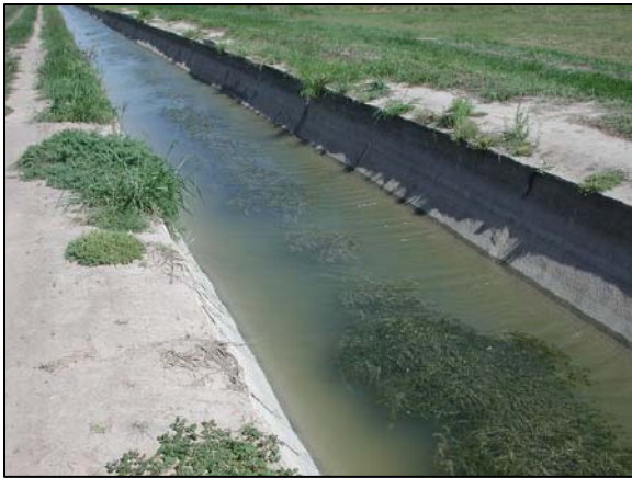
Figure 1. West Main Canal
