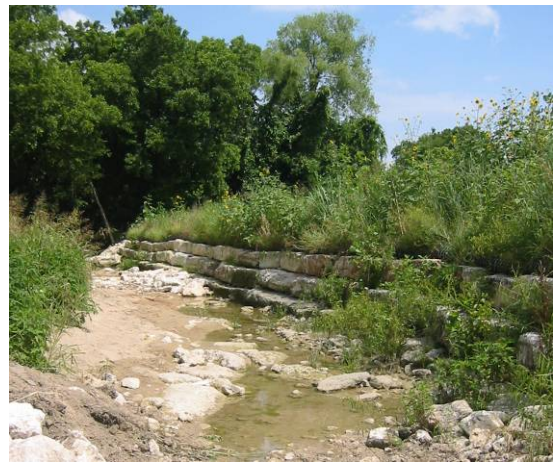
Figure 8. Stream stabilization using limestone boulders and riparian vegetation along the banks
