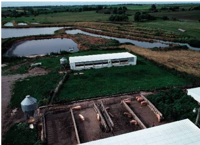
Figure 9. NRCS photo of constructed wetlands used to treat swine farm lagoon effluent
