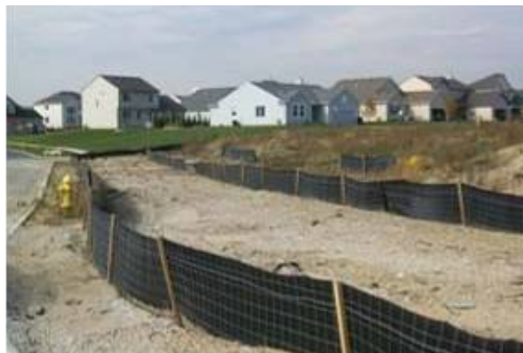
Figure 13. NRCS photo of a silt fence around a construction site
