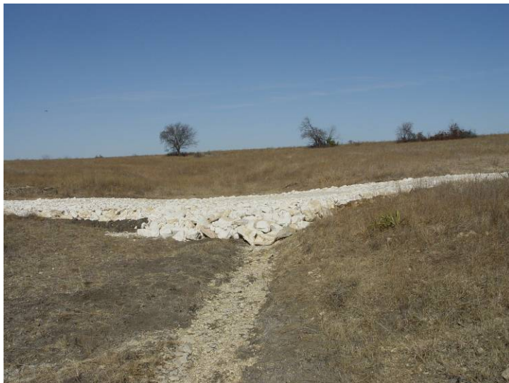
Figure 11. Check dam photo from Ft. Hood re-vegetation project (Courtesy of W. Fox).
