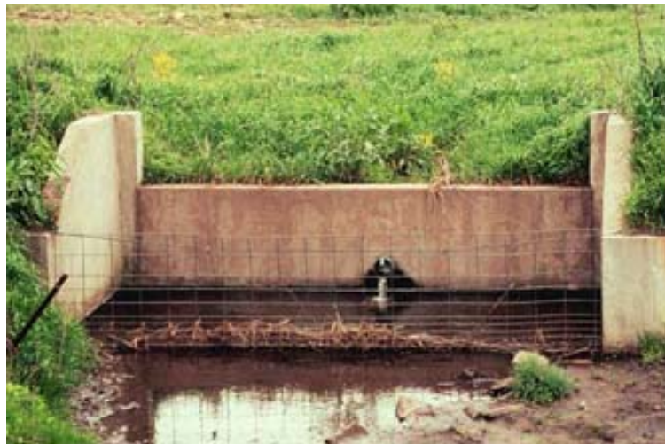
Figure 24. Graded Stabilization Structure
