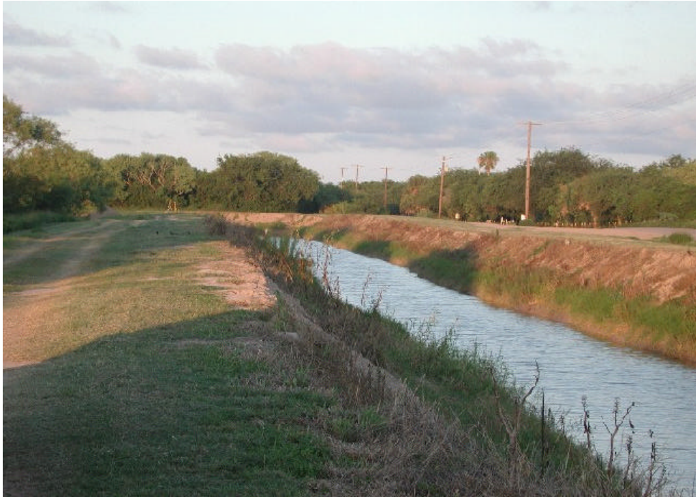
Figure 7. View of the Main Canal Test Segment.
