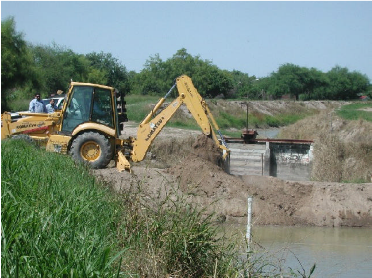
Figure 2. Downstream test dam being removed by the Brownsville Irrigation District.
