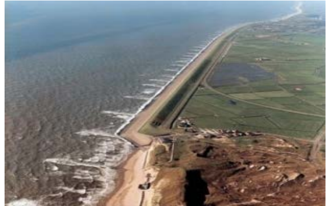
Figure 2: Typical coastal levee (The Netherlands)
