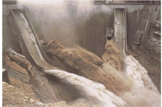
Figure 13: Spillway discharging at the Jiroft dam in Iran
