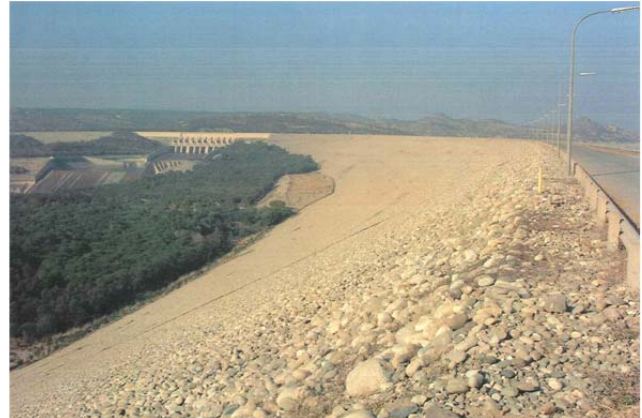
Figure 2: The 148 m-high Mangla dam, Pakistan, completed in 1967 and recently heightened
