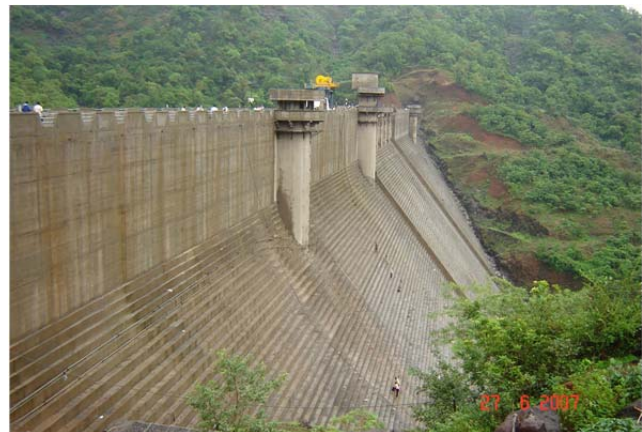
Figure 4: The Lower Ghatghar RCC dam in India, which forms the lower reservoir for a 250 MW pumped-storage scheme
