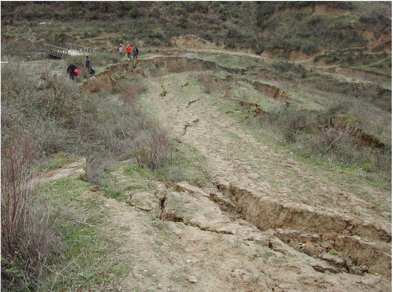
Figure 11: The Sharredushk dam in Albania
