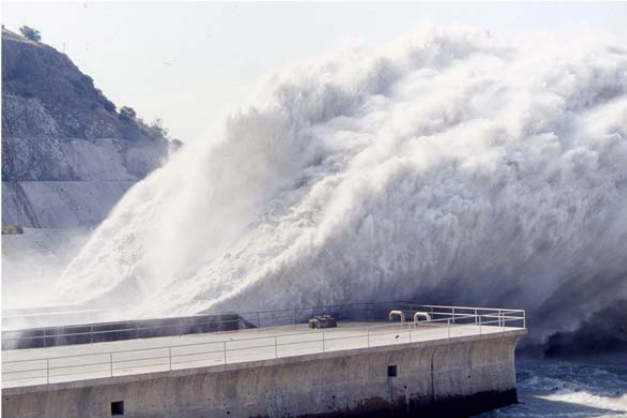
Figure 1: One of the irrigation outlets discharging at the Tarbela dam in Pakistan
