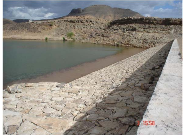
Figure 8: Bani Naji dam in Yemen.
