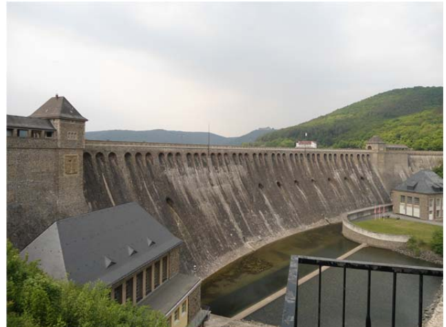
Figure 10: The Eder multipurpose dam in Germany
