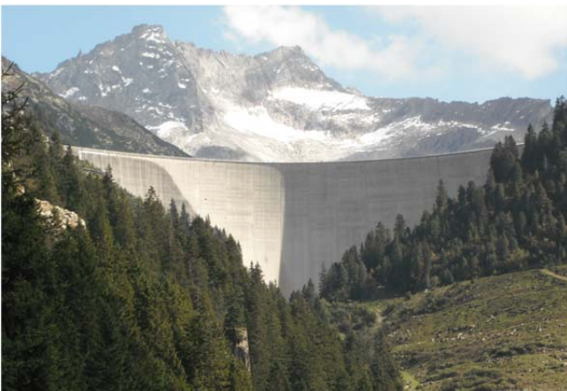
Figure 3: The 186 m-high Zillergründl dam in Austria
