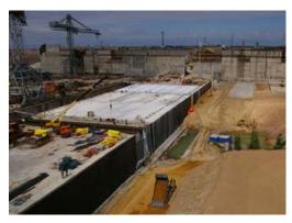
Figure 5: Tunnel construction beneath S1 navigation opening
