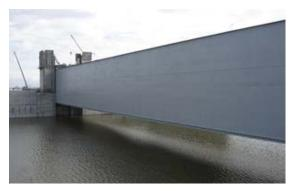
Figure 7: Gate at S2 Navigation Opening (in maintenance position)
