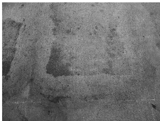
Figure 4. Decontaminated concrete surface
