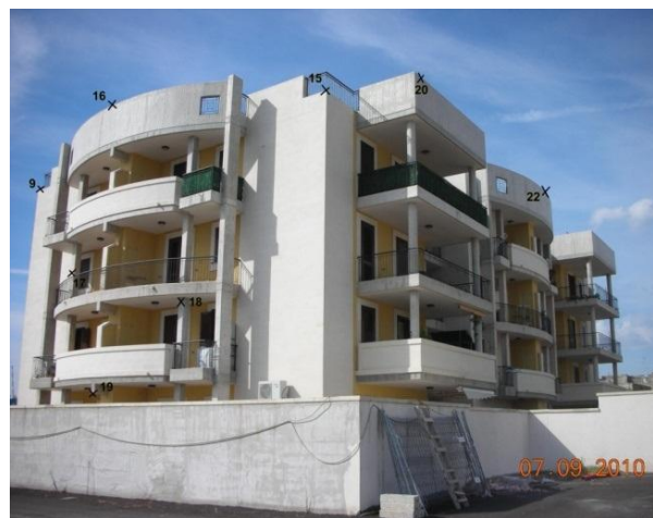
Figure 9. Control vertices located on the South and East sides
