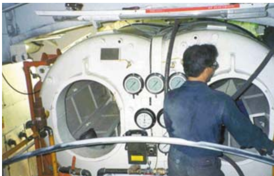
Tunnel boring machine (TBM) lock
