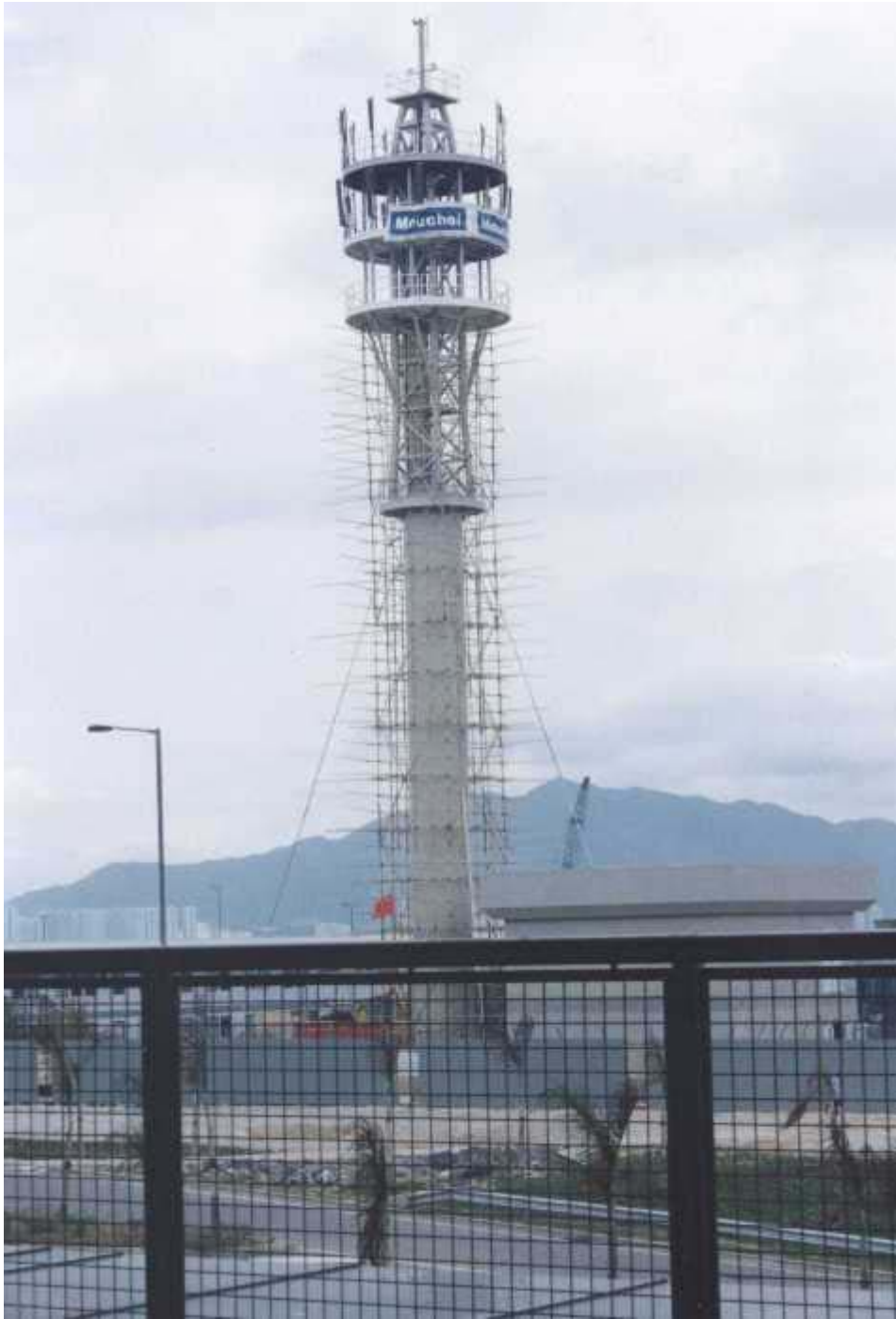
Figure 4.9 Single layered scaffold around a circular tower for access
