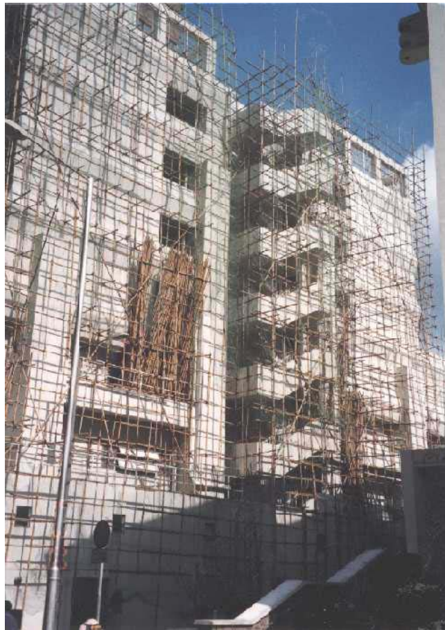
Figure 4.8 Scaffold for renovation work
