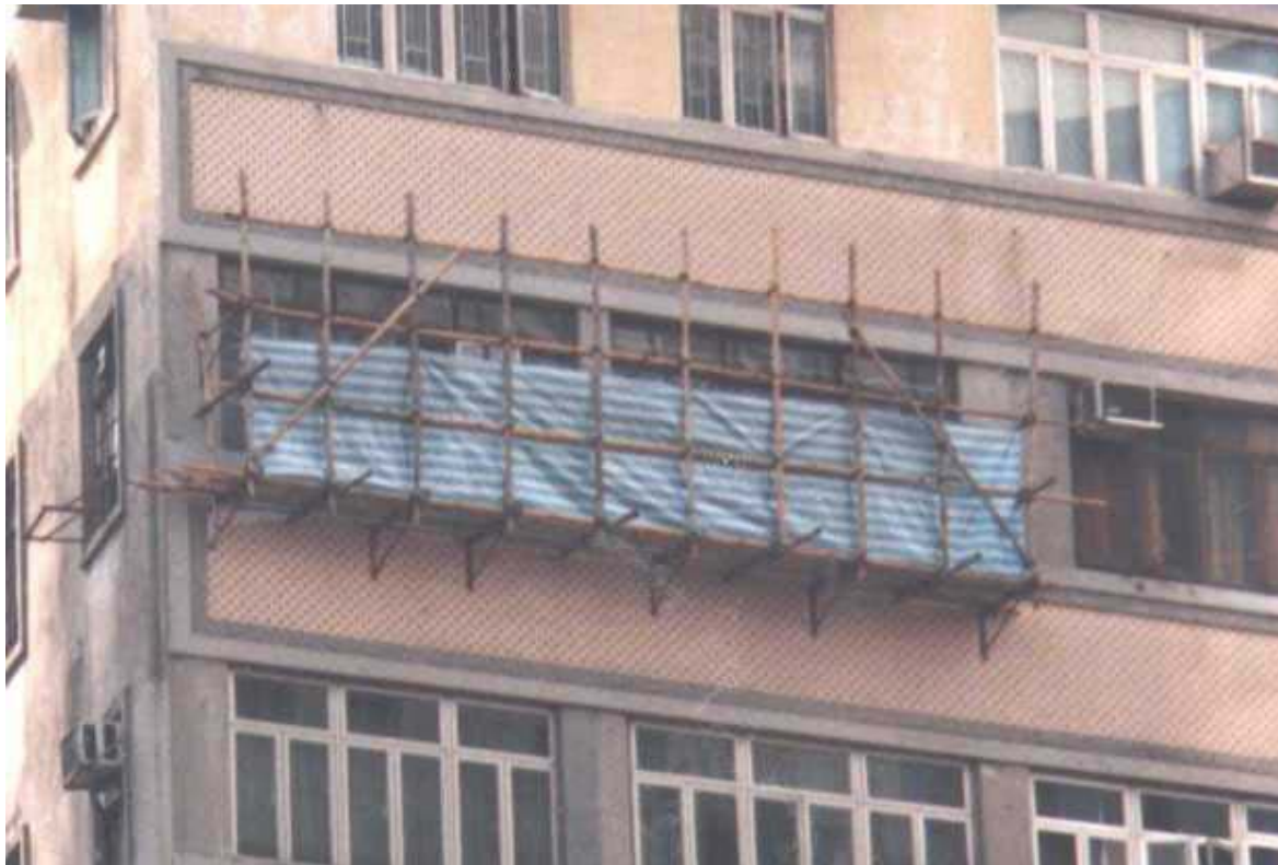
Figure 4.6 Truss-out scaffold for repair of external walls
