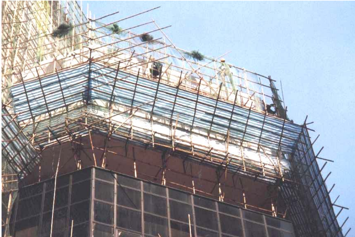
Figure 4.3 Catch fan in double layered scaffold
