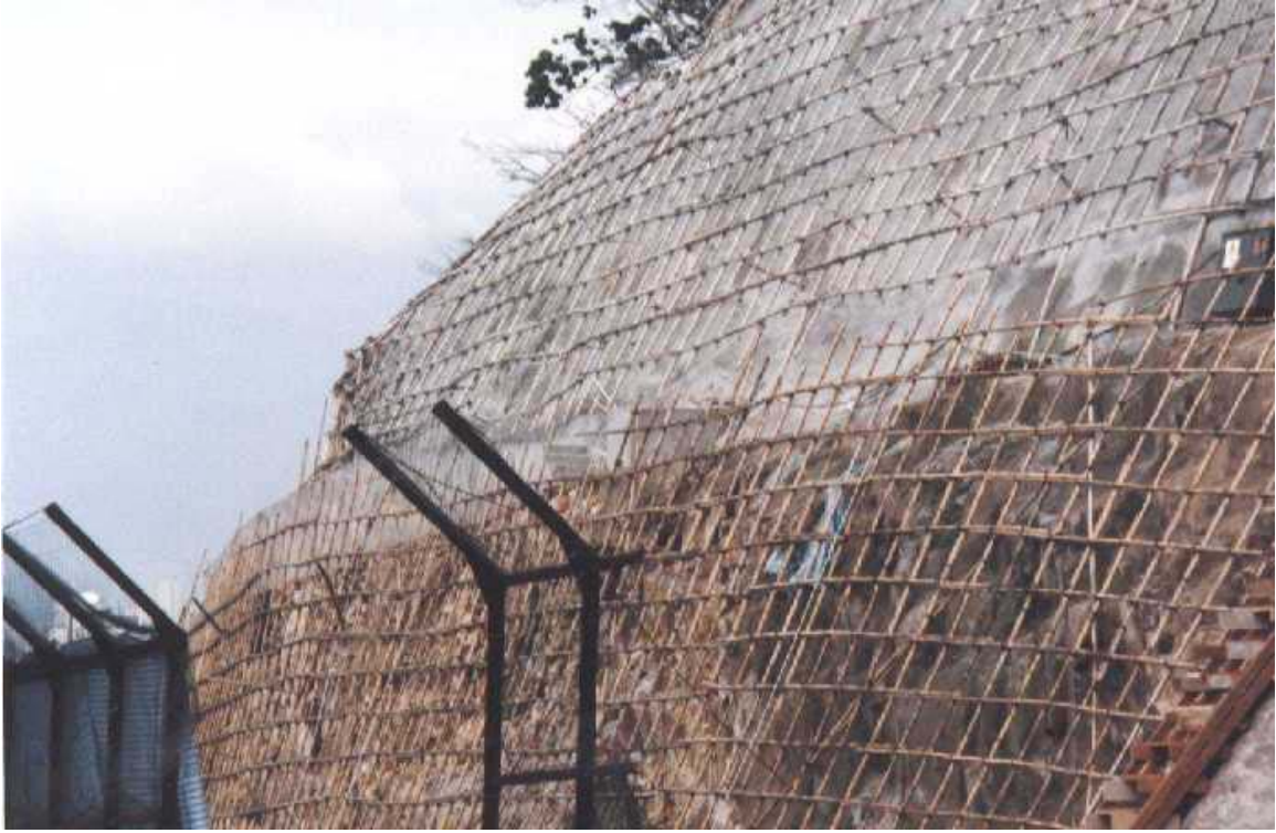
Figure 4.7 Civil work scaffold on slope
