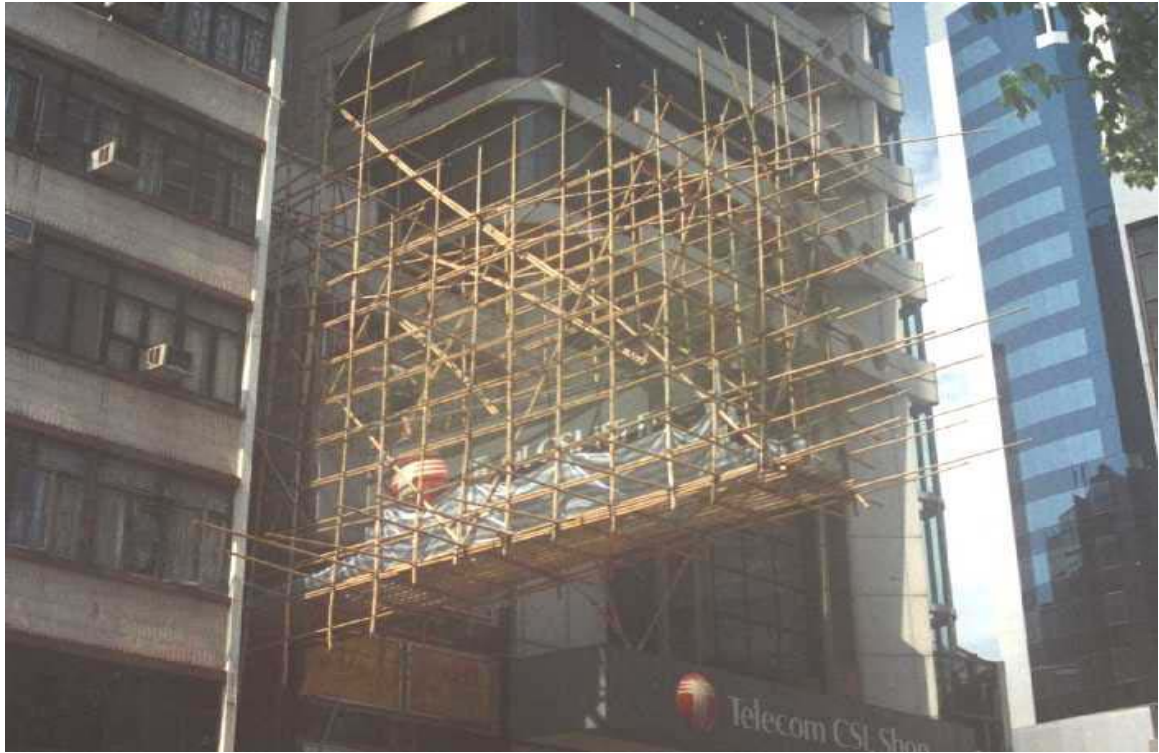
Figure 4.5 Cantilever scaffold for signage work
