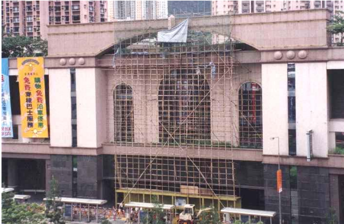
Figure 4.1 Single layered scaffold
