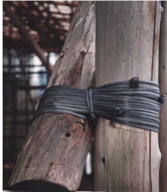
Figure 6.1 Knots in bamboo scaffolds (continued)
