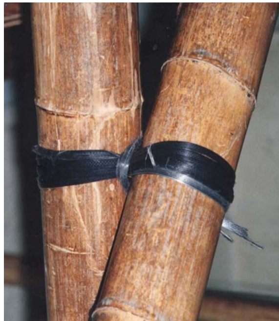
Figure 6.1 Knots in bamboo scaffolds
