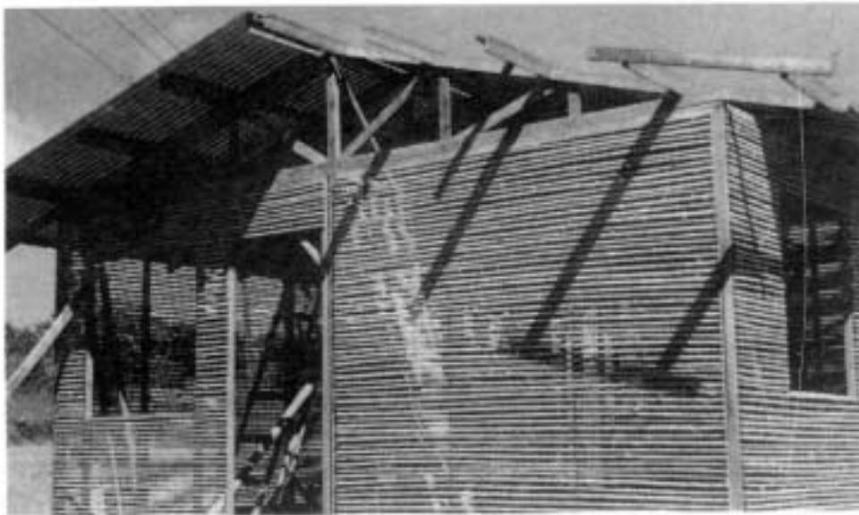
Fig. 19: Bamboo house – internal frame with paneling and corrugated roof
