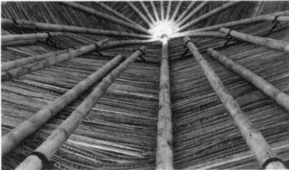
Fig. 4: Guadua bamboo as structural element, El Tapir Restaurant by PNB
