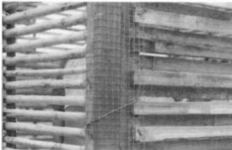
Fig. 9. Cana brava panel (left side) joined with a tablilla panel (right side)
