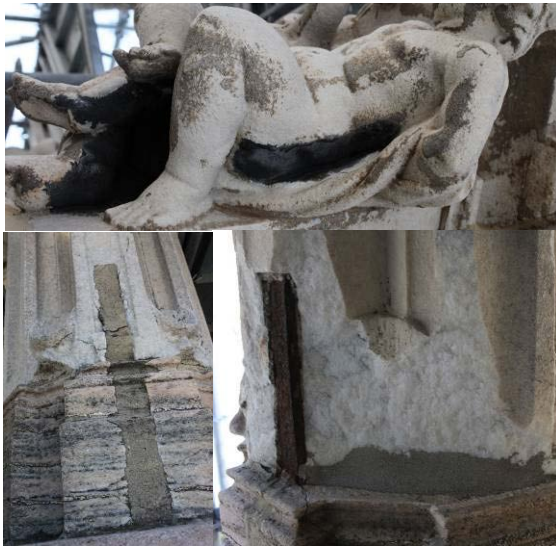
Figure 4: Degradation of marble blocks. In the image above the presence of black crust and artificial patinas. Candoglia marble has a significant pyrite content that may be sporadic or even have large aggregates of crystals. There are also rare grains of magnetite. The presence of metal minerals determines, unfortunately, a lack of durability, with the consequent need for damaged parts to be replaced continuously. Images below show an important detachment of material and deterioration of the old iron anchorage.
