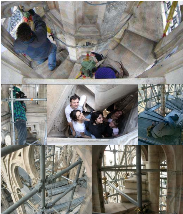
Figure 1: Some fun pictures of survey moments on the spire. The image shows work conditions and the environment to be measured.
