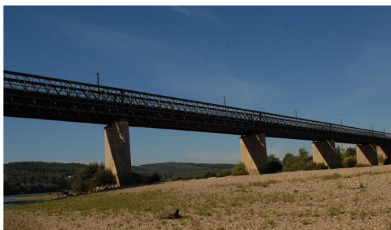
Figure 8. Bridge in Praia do Ribatejo, over Tejo river
