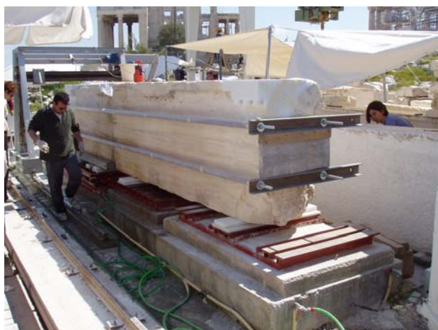
Figure 9. Binding of the beam fragments after the joining
