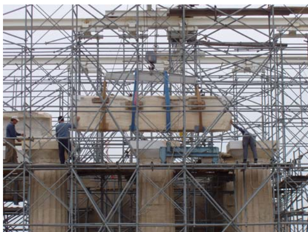
Figure 5. Resetting of a architrave after its structural restoration
