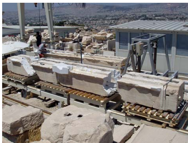
Figure 7. Joining of fragments of a beam by means of titanium bars, at the specially designed table. By T. Tanoulas.
