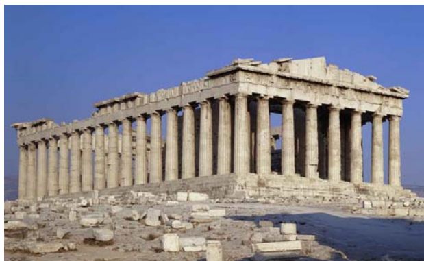
Figure 2. The Parthenon. View from north - west. By S. Mavrommatis
