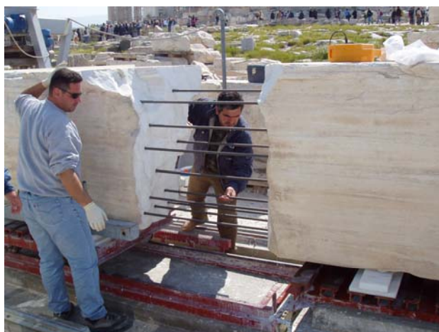
Figure 8. Preparation for the joining of the beam fragments
