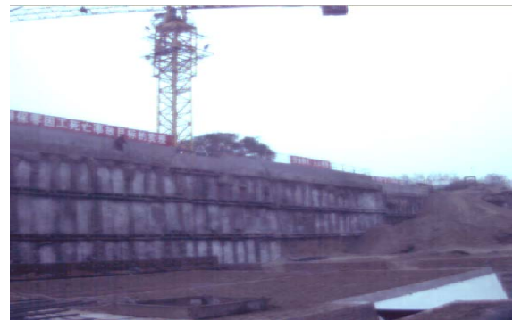
Figure 7. The side slope of metro in shenyang
