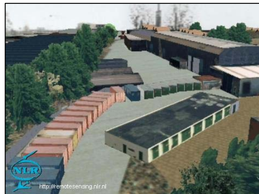
Figure 4. A 3D visual reconstruction of the central bunker complex surrounded by containers at the SE Fireworks premises.
