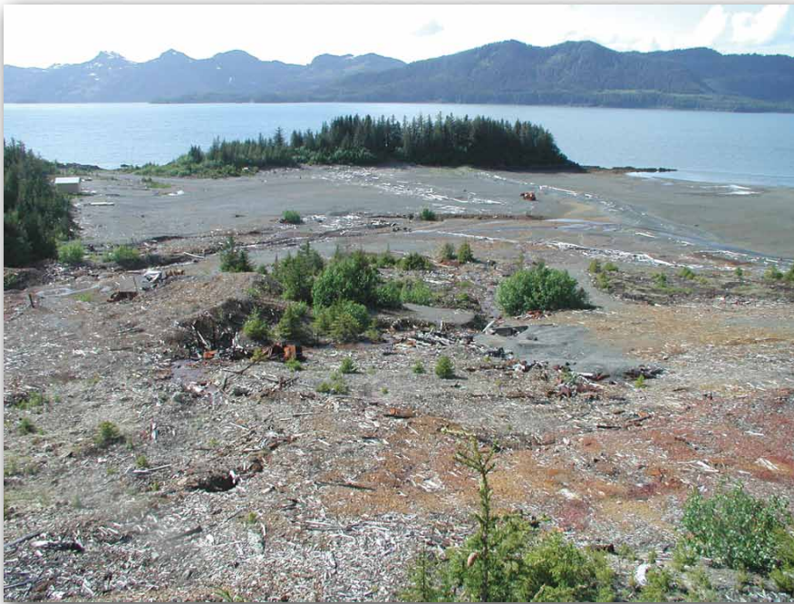
Figure 3. View westward across degraded sulfide-bearing waste rocks at the Beatson mine site, Alaska. Erosion and oxidation of the waste piles result in dispersal of sulfide particles and dissolved metals into Prince William Sound. Copper was mined from the Beatson deposit between 1904 and 1930.
