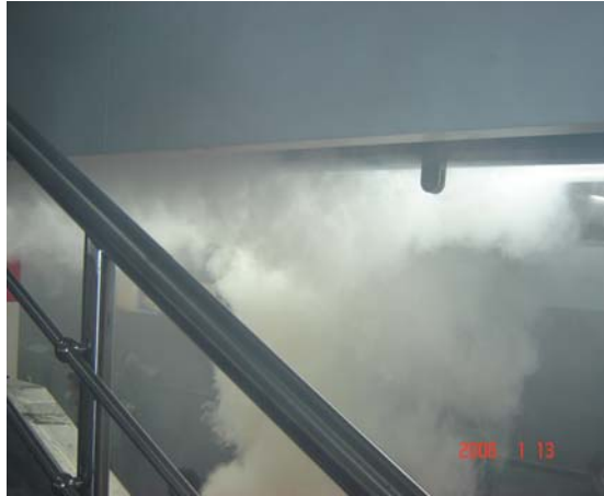
Fig.5. status at the mouth of the escalator under platform cold smoke test (cold smoke source was in the mouth of escalator)
