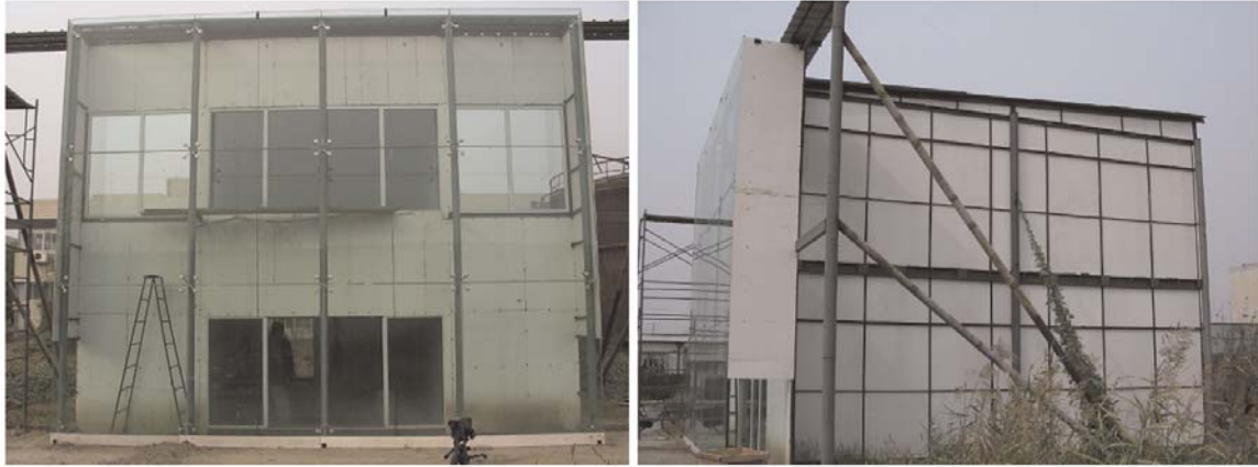
Figure 1 Two-storey test rig.
