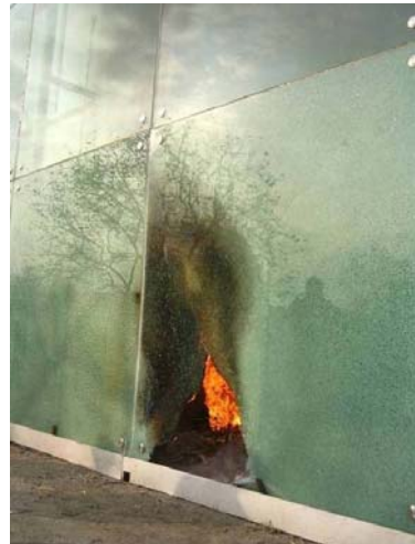
(d)breaking of the external skin glazing
