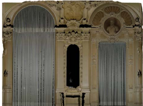
Fig. 9 – The true orthophoto of the western wall.
