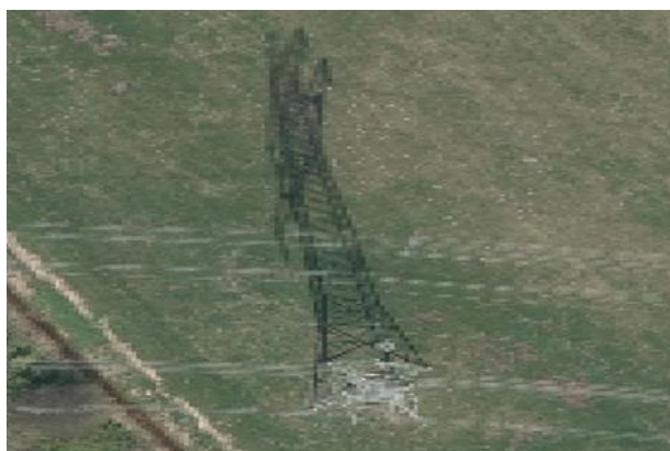
Figure 19. TrueDOP presentation of an electricity pylon
