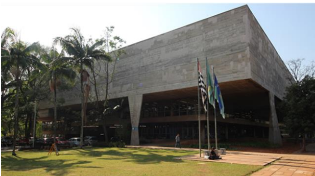
Figure 1. External view of the FAU USP building
