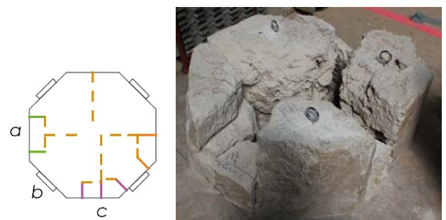
Figure 10. Pillar n. 12 – row I. On the left, diagnostic drawing; on the right the ashlars disassemble and reassemble on the floor of the Basilica.
