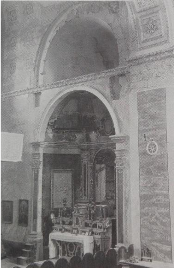
Figure 3. The altar of the Holy Heart of Mary still in situ, before the dismantling, in the left apse of Gerace Cathedral (1934).
